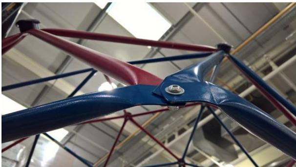
**Figure 29. Flattened metallic tube, angled, bolted joint**
