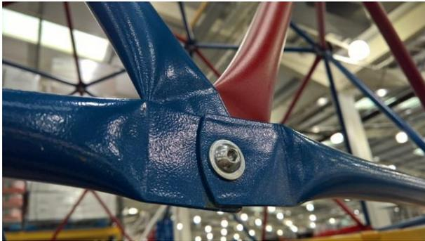
**Figure 28. Flattened metallic tube, bolted joint**
